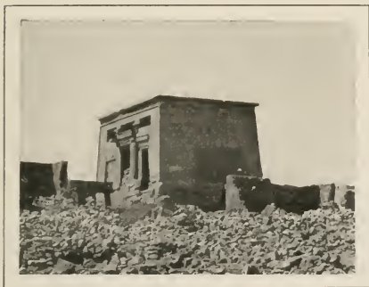
FIG. 443.—TEMPLE OF TAFEH BEFORE RESTORATION. (Phot. E. Brugsch.)
